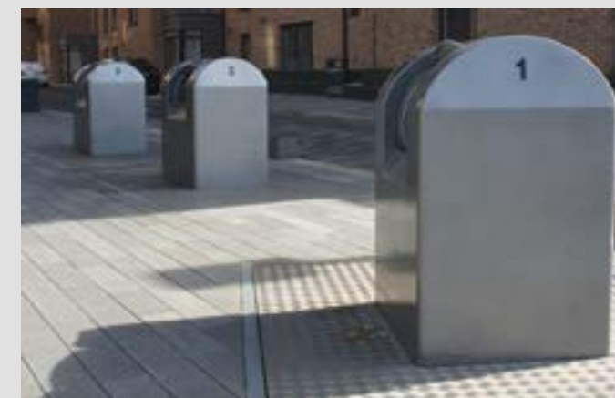
Underground bins for residual waste allow large volumes to be held with minimal impact on the street scene. It is important that the Council's Waste and Cleansing Service are involved early, as their requirements may impact on the design.
