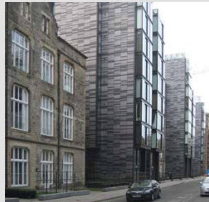
Aluminium—Simpson Loan Multi-toned anodised aluminium cladding provides a striking and positive contrast to the historic buildings making the distinction between new and old very clear.
