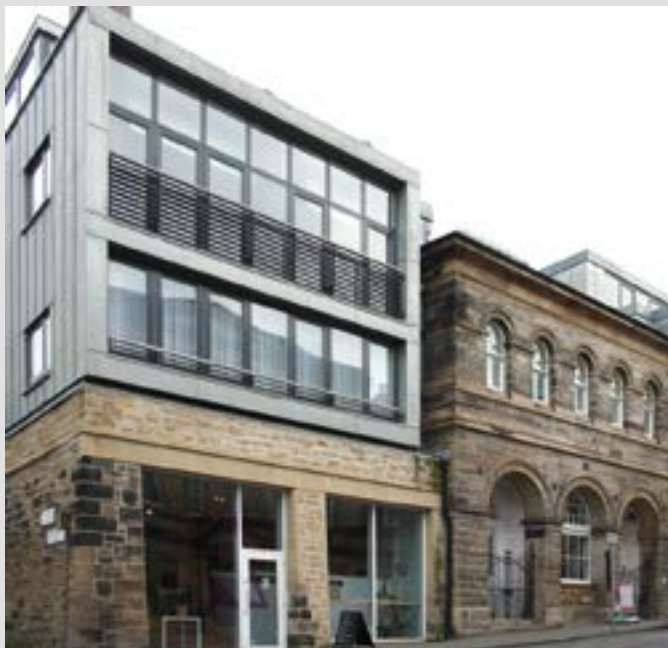
Using zinc to provide striking contrast—Infirmary St. The zinc cladding combined with the modern building form provides a positive contemporary contrast to the historic former Infirmary Street Baths building.
