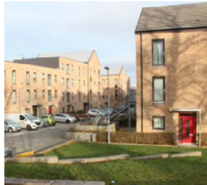
Terraced slopes and shared surface 'home zone' street at Gracemount.
