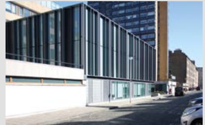
Curtain Walling—Beccleuch Place The potential offered by glazing systems with variations in the window widths, patterning of the glass and mullion depths is fully taken advantage of here.
