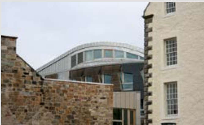
Metal roofing in a historic context—Canongate Stainless Steel roofing has been used on the Scottish Parliament.
