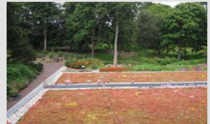
Extensively green roof—Botanic Gardens The planting on this green roof helps integrate the building into its surroundings.
