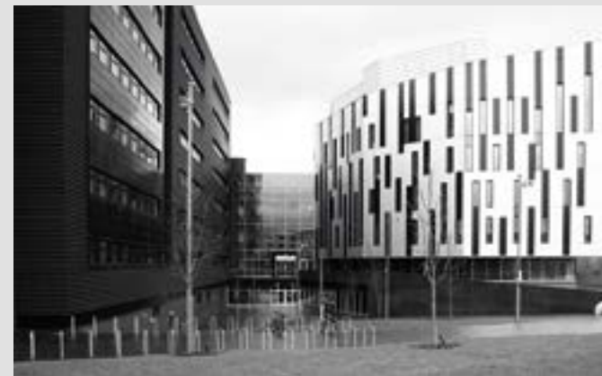
High quality detailing—Sighthill Court Construction of a sample panel and approval were required by condition in order to ensure the design intent of a high quality finish was executed.
