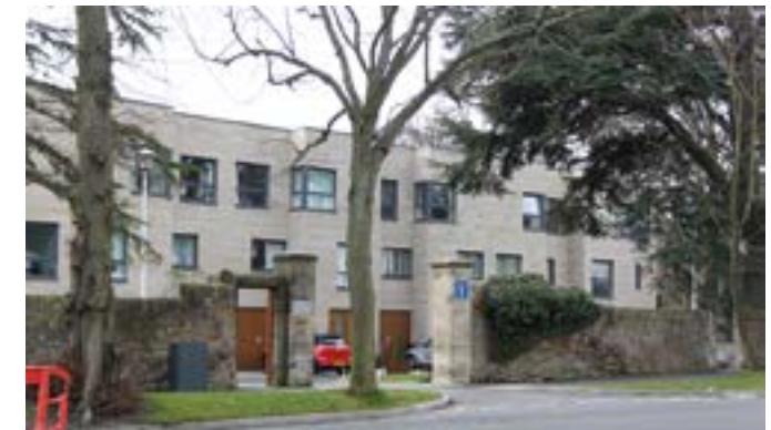
Boundary walls in villa areas—Newbattle Terrace Boundary walls are extremely important to the character and appearance of villa areas. The size and number of new openings to them should be minimised.
