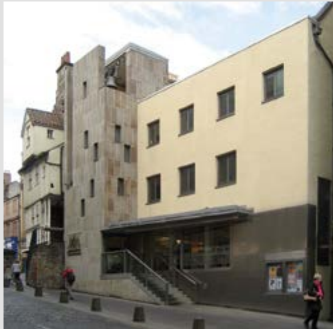
Integrating the new with the old—High Street
