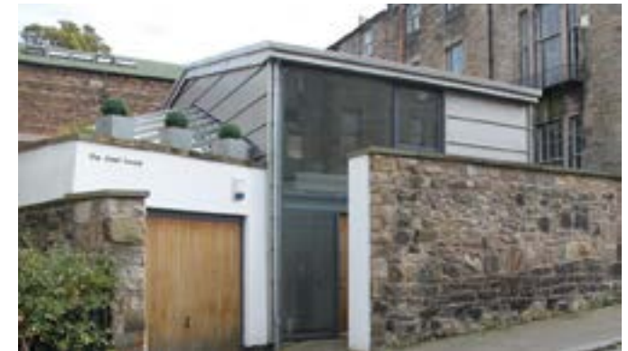
Incorporating a boundary wall—Hart Street This stone wall was re-used and incorporated into the new house.
