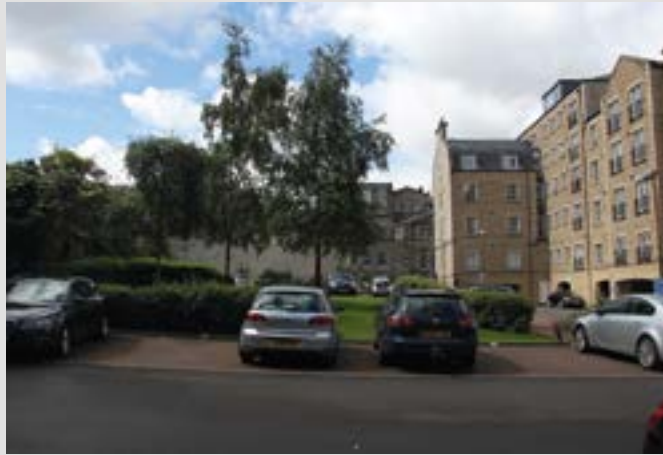
Rear courtyard parking within well overlooked landscaped amenity space off Gayfield Square
