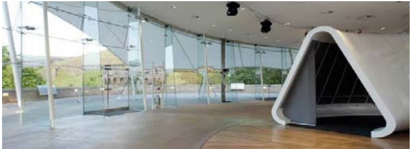
Good design for noise was used at Our Dynamic Earth to stop noise escaping from one of their function areas. Instead of installing doors they installed a triangle, zigzagged corridor.
